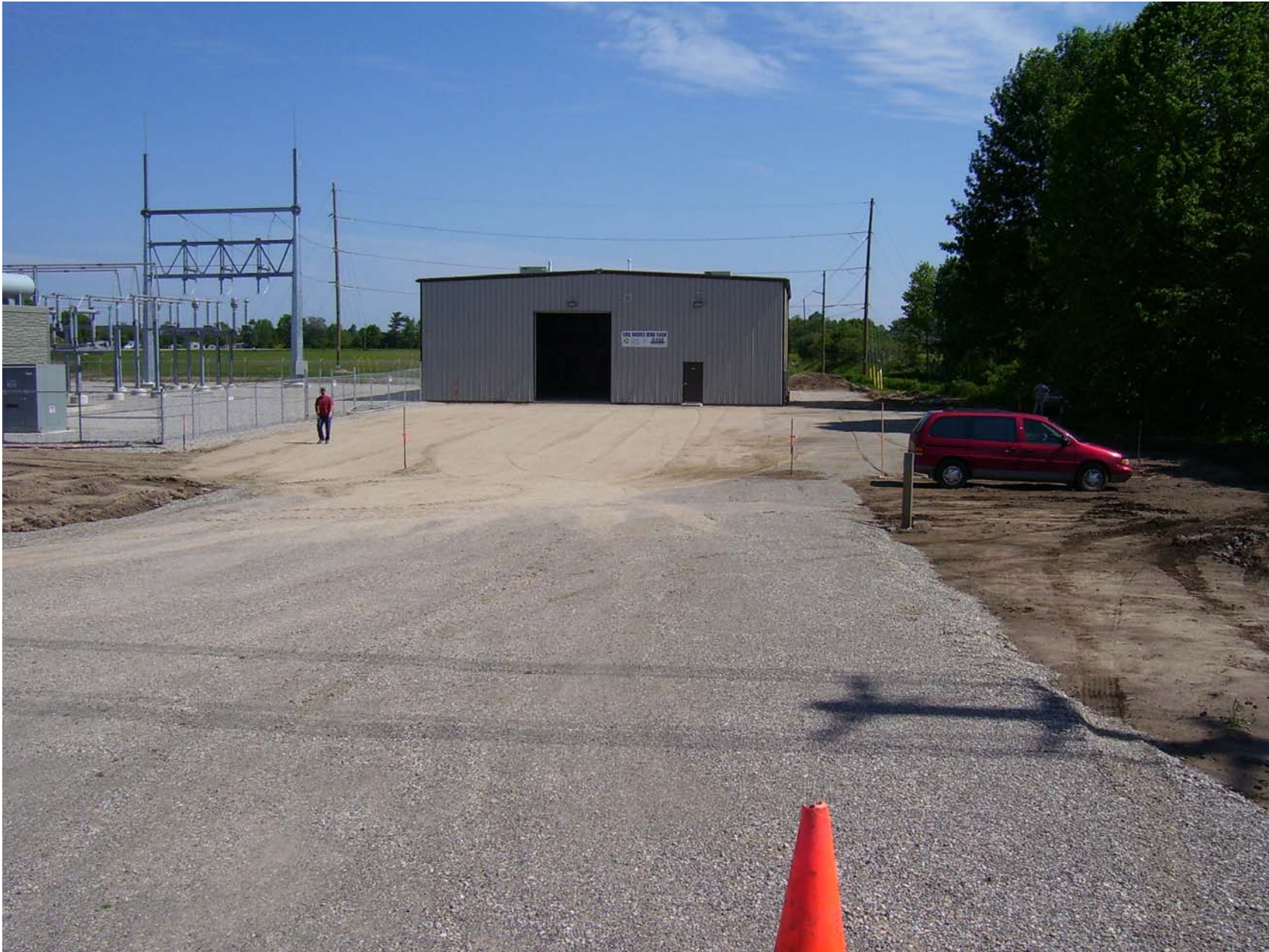
Figure 2-26. Photograph of Representative Service Building
